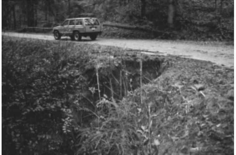
*Sedimentation from unimproved and gravel roads can be reduced when best management practices, such as grassed road shoulders and rip-rap, are installed properly and well maintained.*
