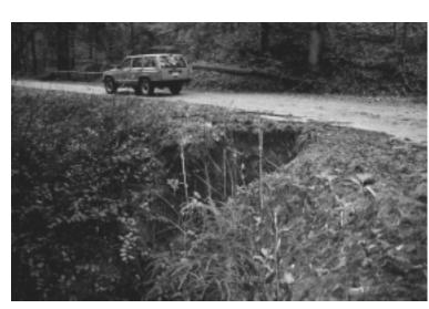
Sedimentation from unimproved and gravel roads can be reduced when best management practices, such as grassed road shoulders and rip-rap, are installed properly and well maintained.
